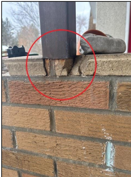
Cracked bricks
