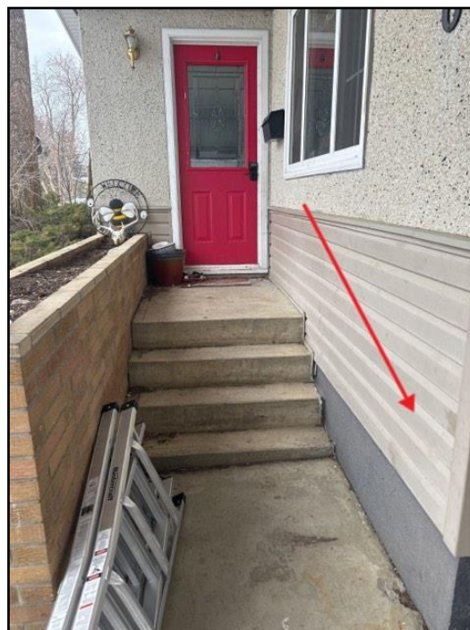
Missing handrail
