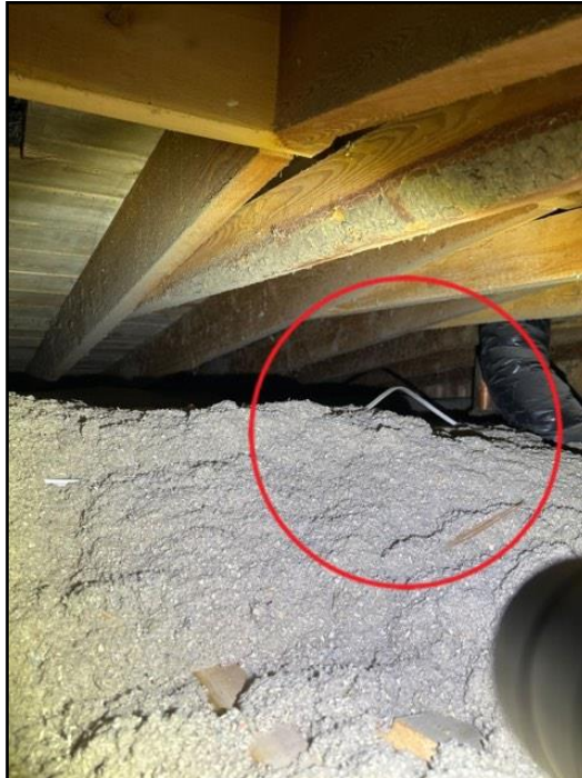
Exposed in attics
