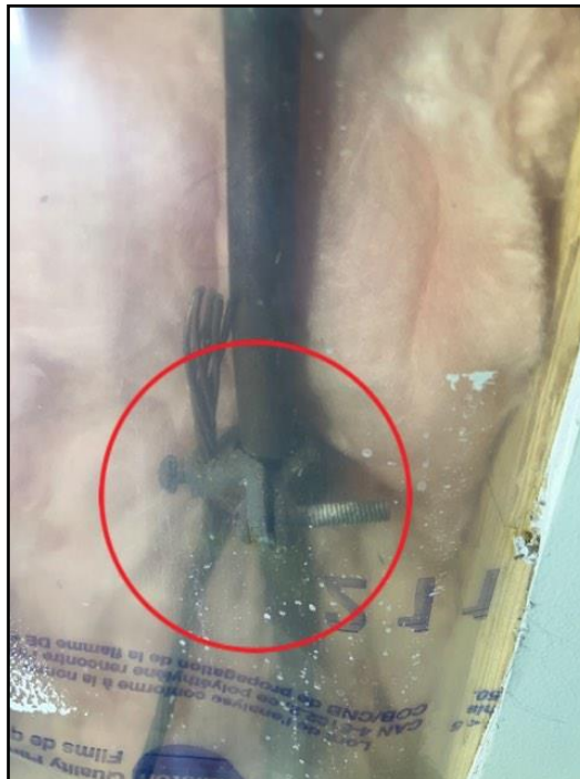
Copper - water pipe
