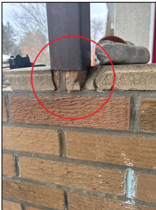
Cracked bricks
