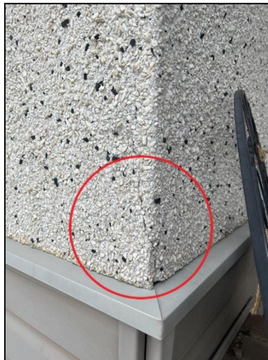
Minor cracks
