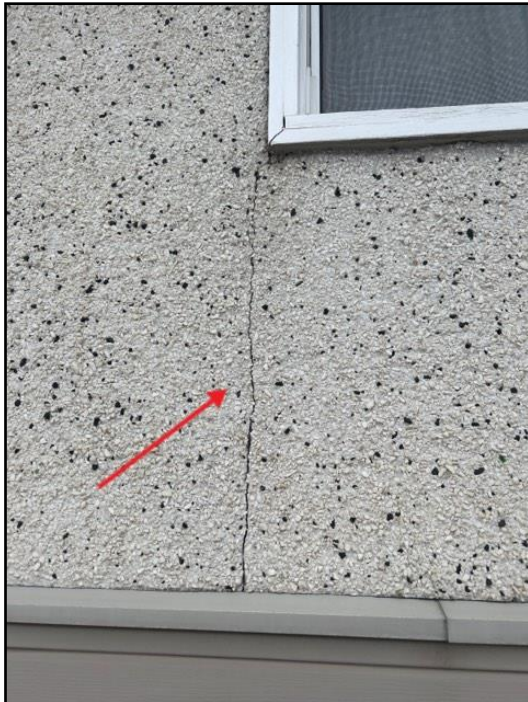
Minor cracks
