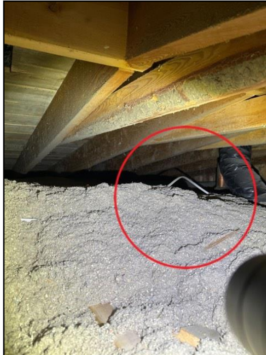
Exposed in attics
