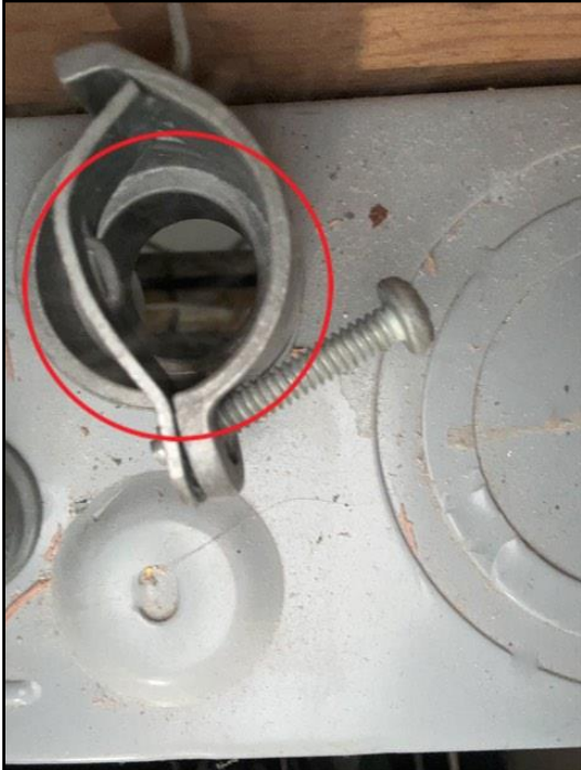
Unprotected openings
